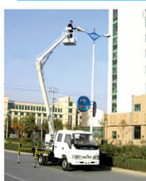
24m Boom Truck Lift
